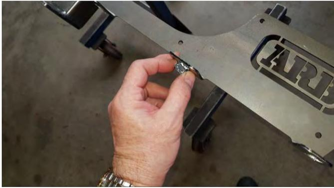
5. Clip M8 cage nuts into all slots. Ensure they can slide freely.
